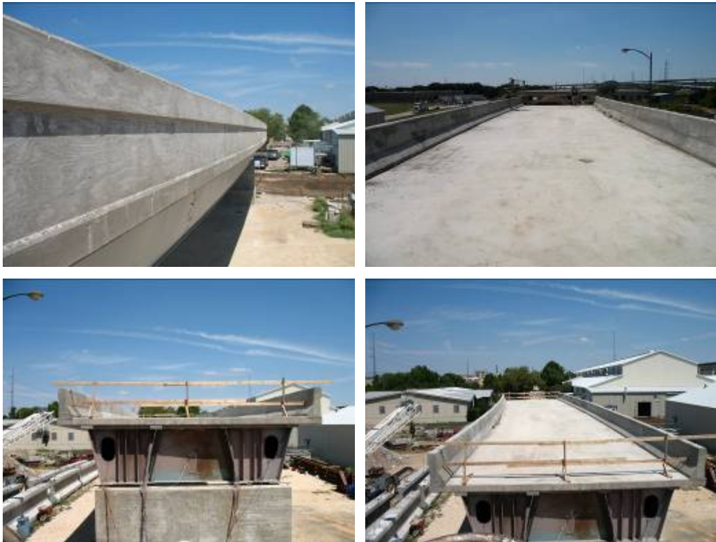
Figure D.10-2: Rails after forms were removed
