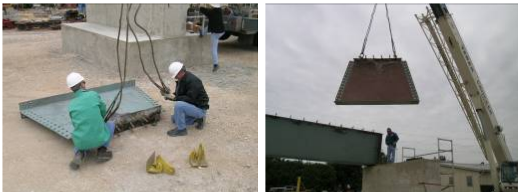
Figure D.2-1: North diaphragm placement
