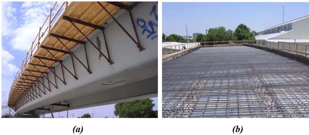
Figure 5.12: a) Formwork on bridge b) deck reinforcing steel
