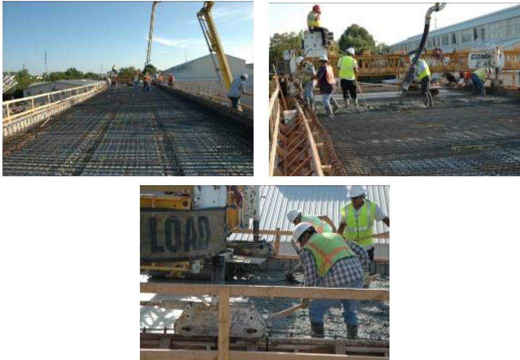
Figure D.9-1: Deck casting starting from the north end using screen
