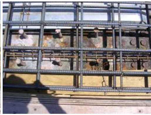
Figure D.7-2: a) Permanent metal decking installation b) edge built up for proper haunch height
