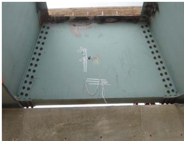
Figure 4.5: Inside of the north end diaphragm
