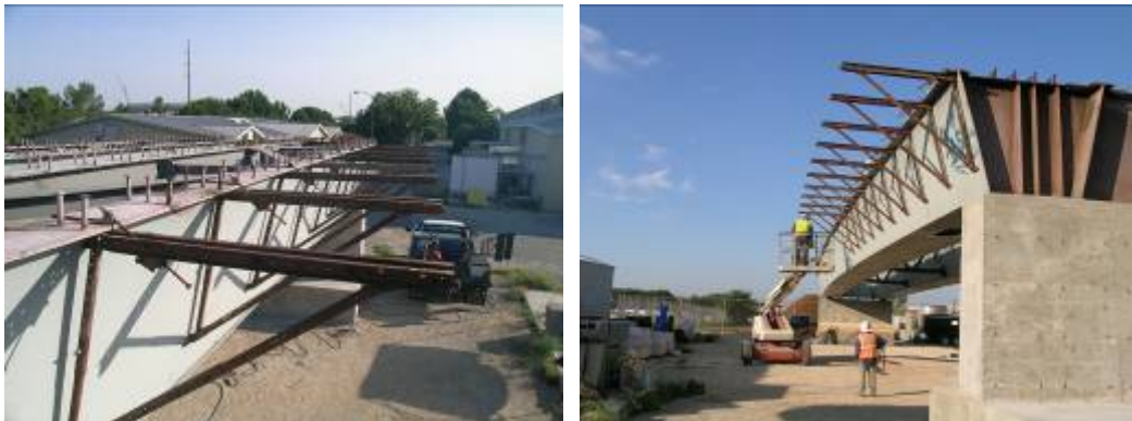
Figure D.7-1: Bracket placement on the girders
