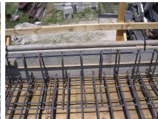
Figure D.7-3: Deck reinforcing steel placement
