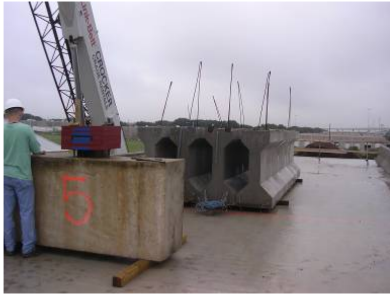
Figure D.12-6: Position 3 during live load testing and the final position for fracture testing
