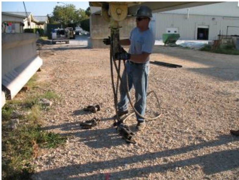
Figure D.12-2: Cables with load cell attached are placed on the crane hook
