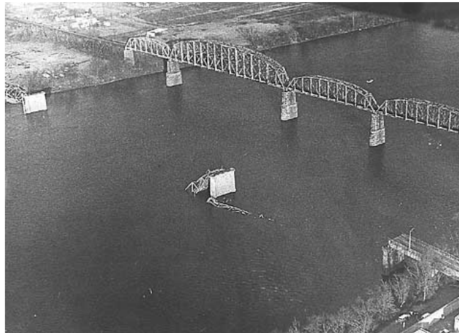
Figure 2.1: Aftermath of the Silver Bridge collapse (Charleston Daily Mail, 2006)
