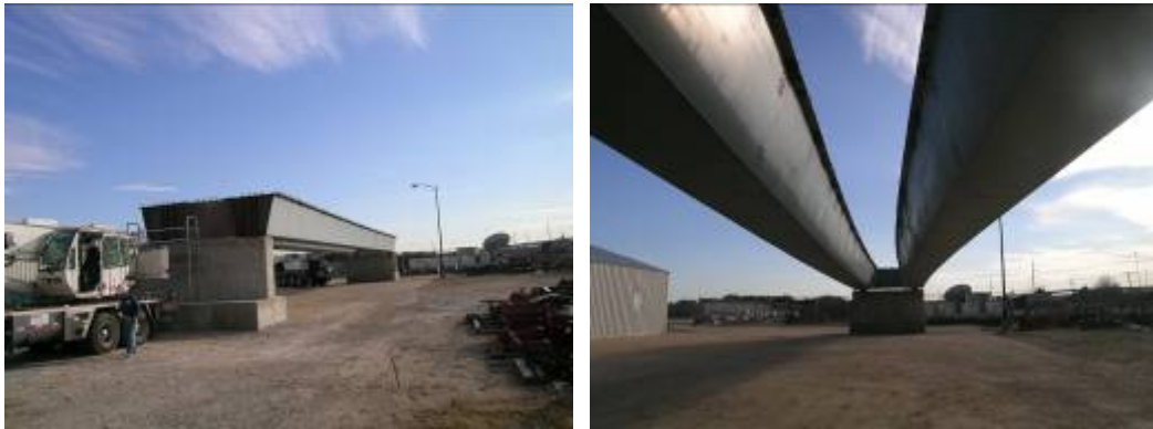
Figure D.2-5: Girders in place on foundations
