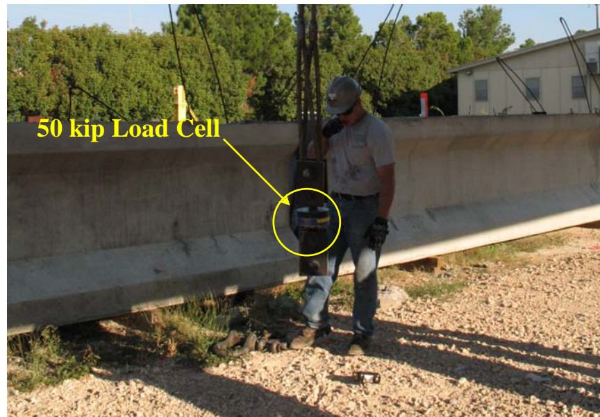
Figure 5.16: Load cell connection to crane
