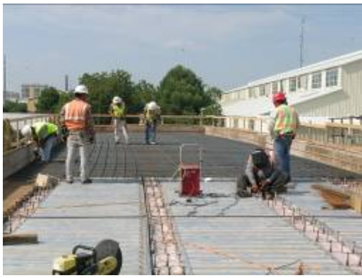
Figure D.7-2: a) Permanent metal decking installation b) edge built up for proper haunch height
