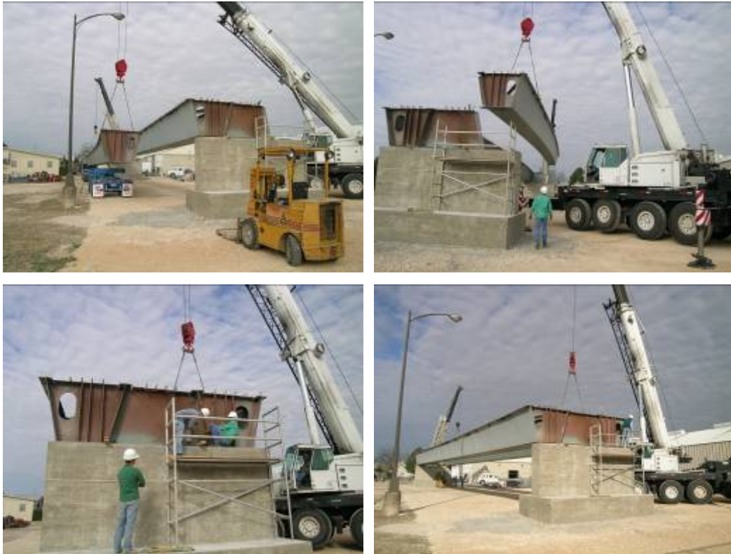
Figure D.2-4: Exterior girder placement
