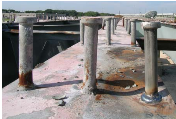
Figure 3.3: New stud welded on to the inner flange of the interior girder
