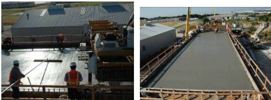
Figure D.9-2: Contractor provided a broom finish
