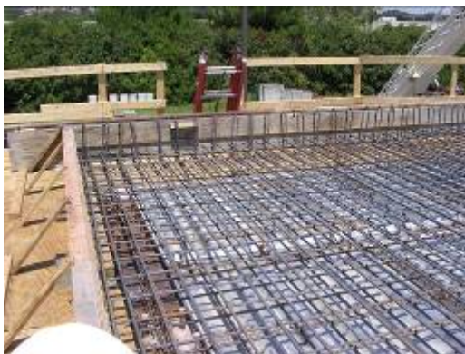
Figure D.7-3: Deck reinforcing steel placement
