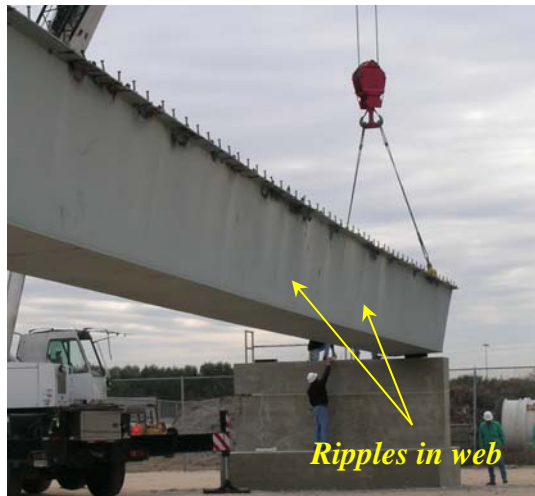
Figure 4.1: Out-of-plane imperfections in the web
