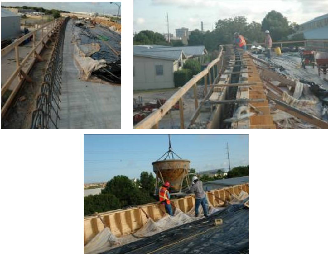
Figure D.10-1: Rail construction
