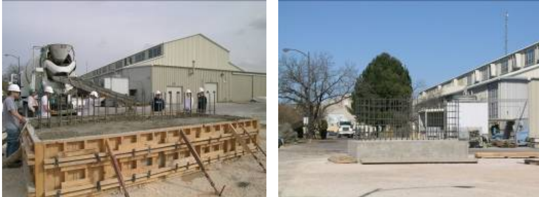
Figure D.1-1: North foundation base
