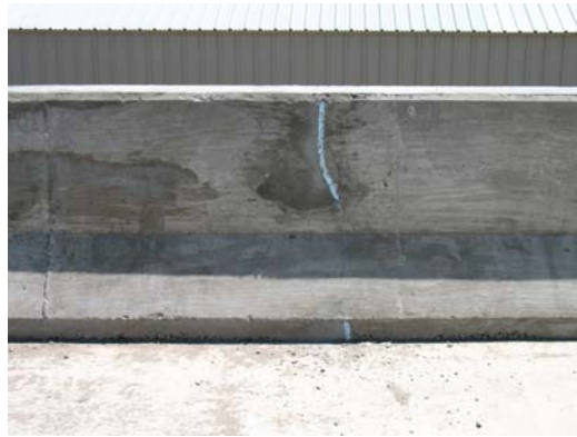
Figure 3.13: Center construction joint on the east rail at midspan
