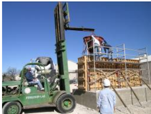
Figure D.1-2: South foundation stem wall
