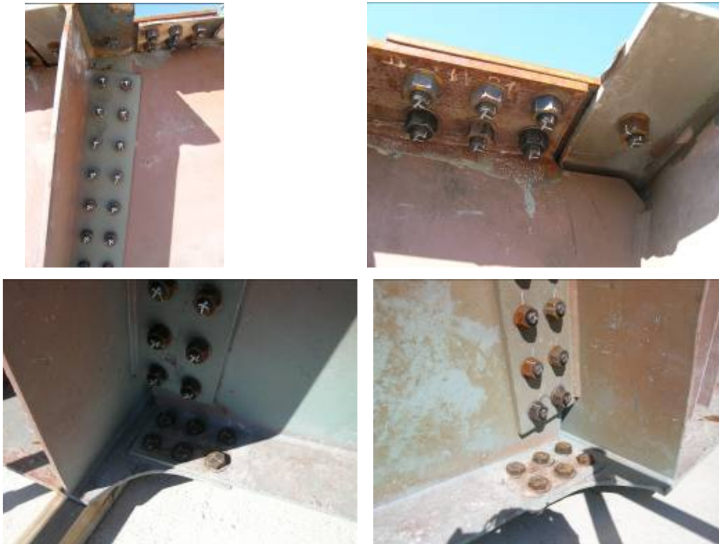
Figure D.3: Diaphragm bolted connections
