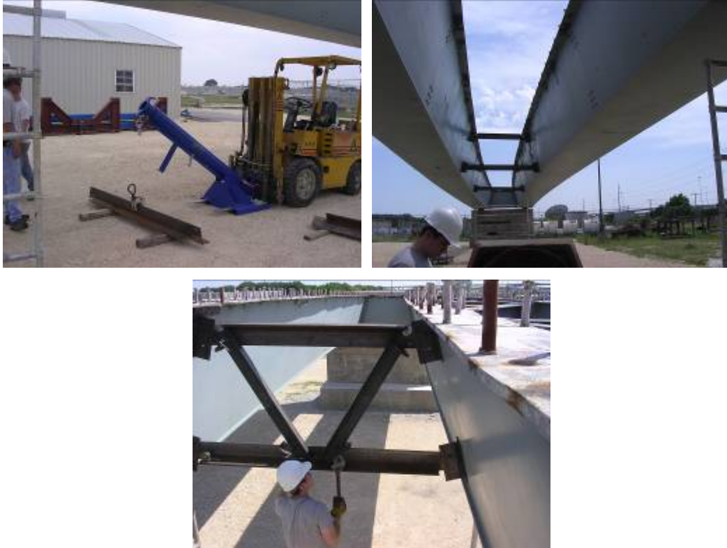
Figure D.4: Bracing installation
