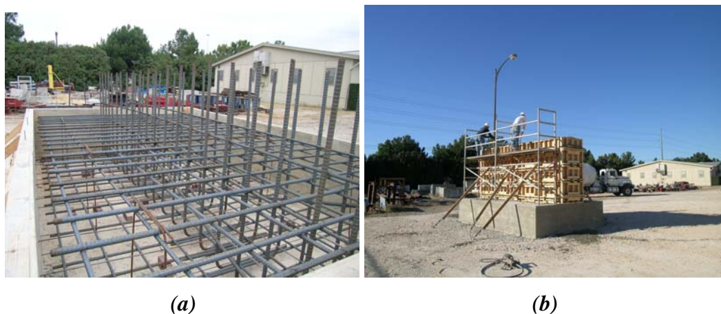
Figure 3.5: a) Bottom of north foundation b) stem wall for south foundation
