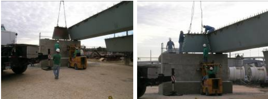
Figure D.2-3: South diaphragm placement
