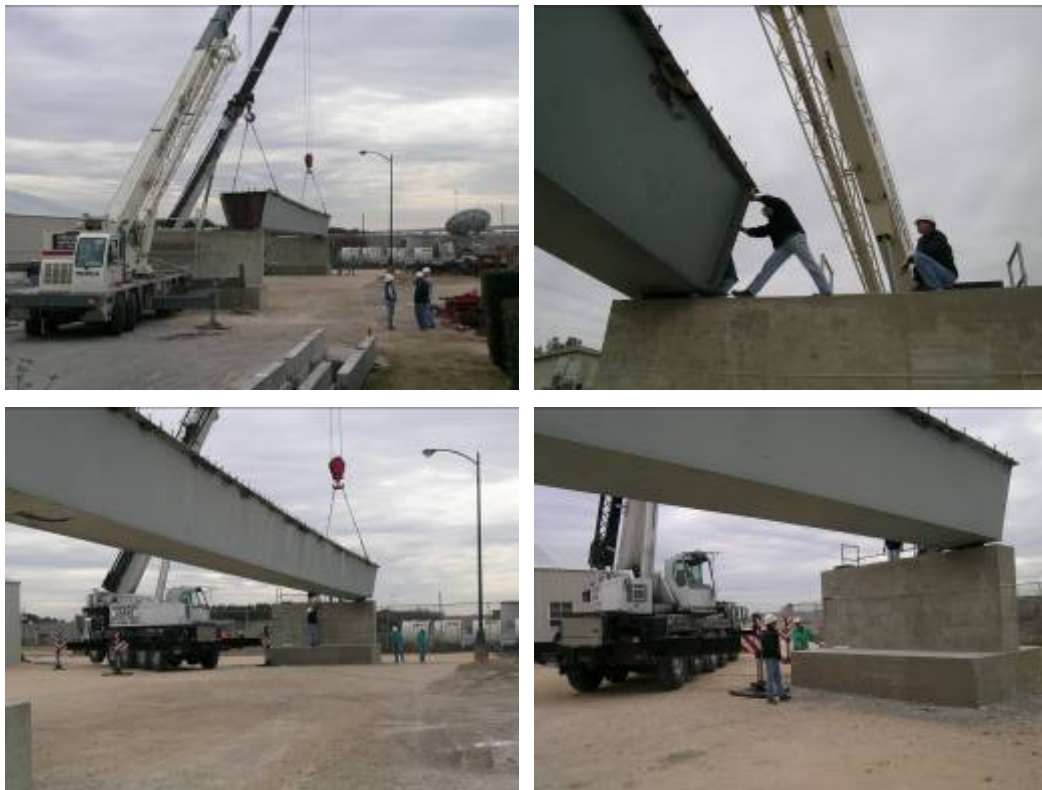
Figure D.2-1: Interior girder placement
